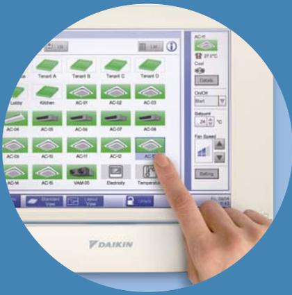
Various types of equipment in a building can be controlled by a single controller.
